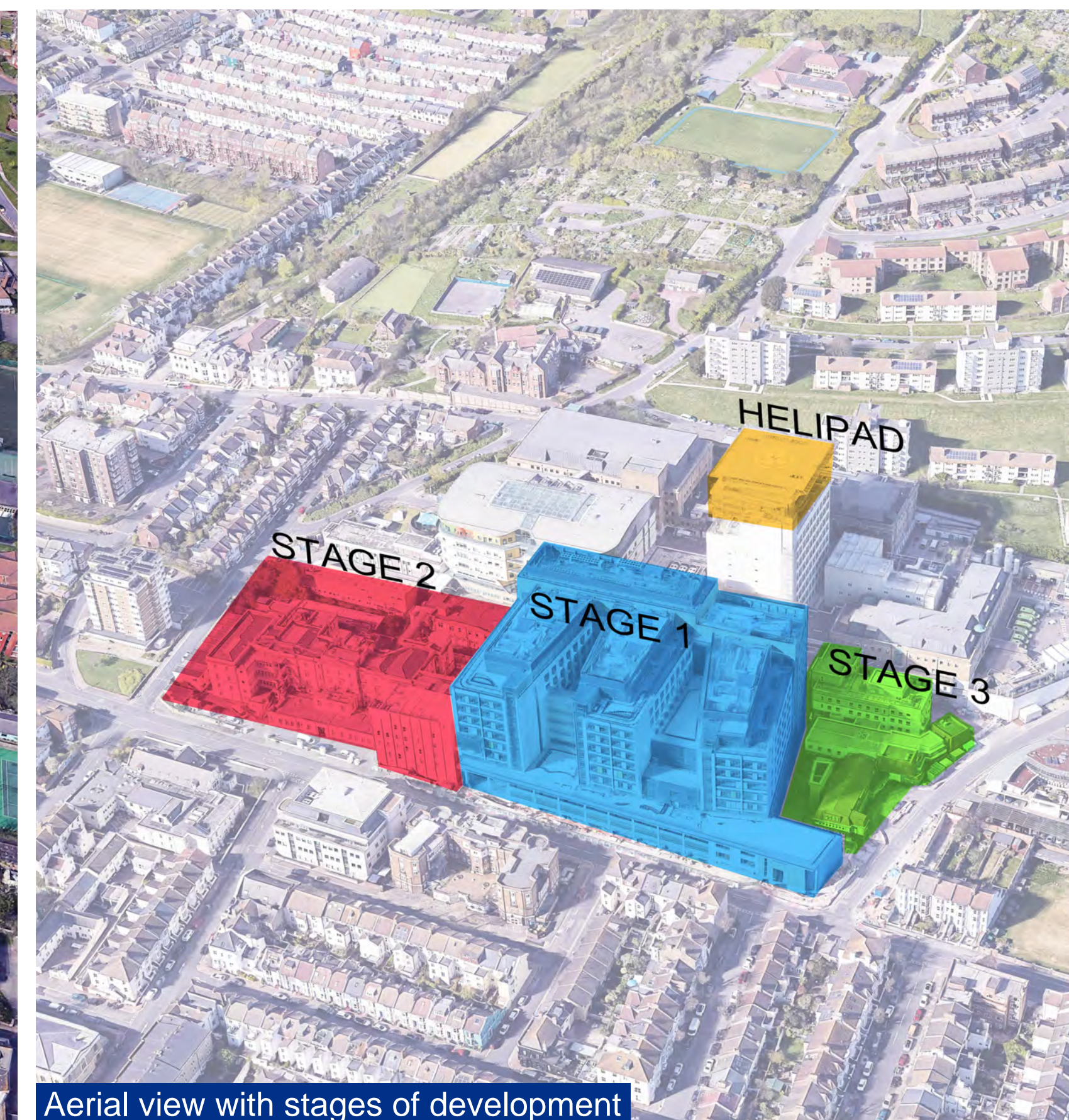
Aerial view with stages of development
