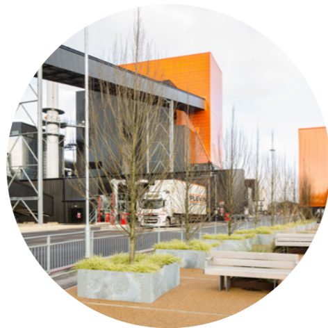
2. Blackburn Meadows Biomass Plant
