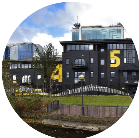
1. Salford Quays Boat Shed
