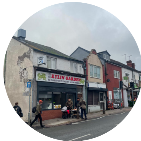
Other buildings are poorly maintained and in need of some repair works
