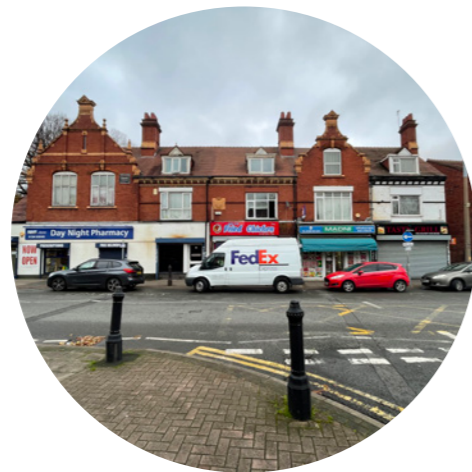
The architectural quality of the upper floors of buildings competes with poorer quality ground floor shopfronts, closed shutters and signage
